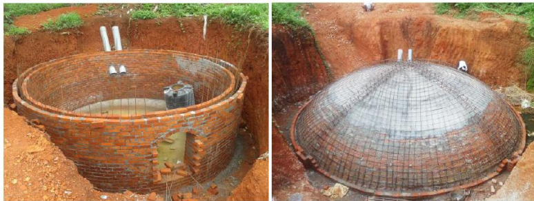
Food and Toilet wastes based Hybrid Biogas plant under construction
