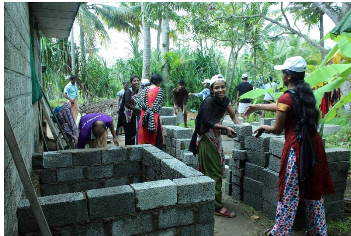
WSE workers engaged in toilet construction
