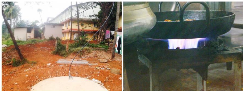
Food and Toilet wastes based Hybrid Biogas plant under working
