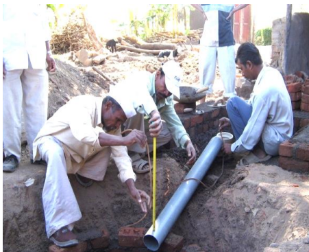
The pipe should have adequate slope
