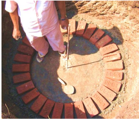
The first layer in 9" Brickwork
