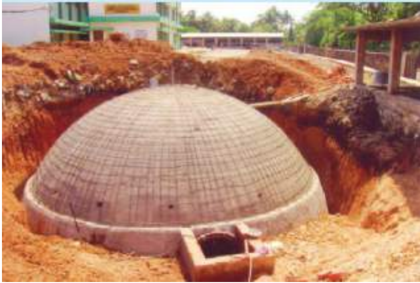
Fixed dome biogas plants
