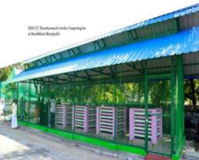
Aerobic bin composting unit (Thumboormuzhi model)
